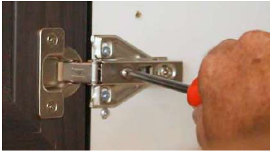
Front screw adjusts door right and left.
