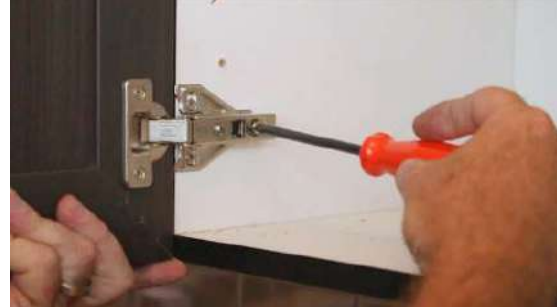
Back screw adjusts door in and out.
