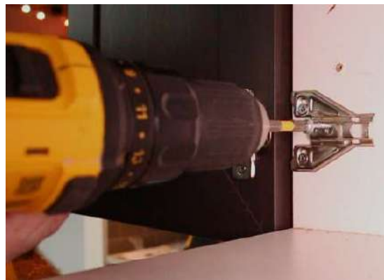
You can screw through the hinge arm. No need to remove it.
